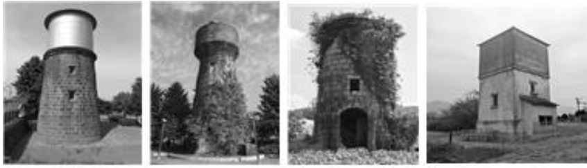
Figure 4 Yeonsan Station(1911), Yeonchun Station(1914), Shinhyunglee(1920), Chupoongryung(1939) Water Towers
